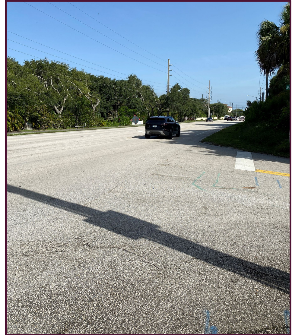
Northbound SR-A1A at the intersection of Jasmine Lane (pre-construction)
