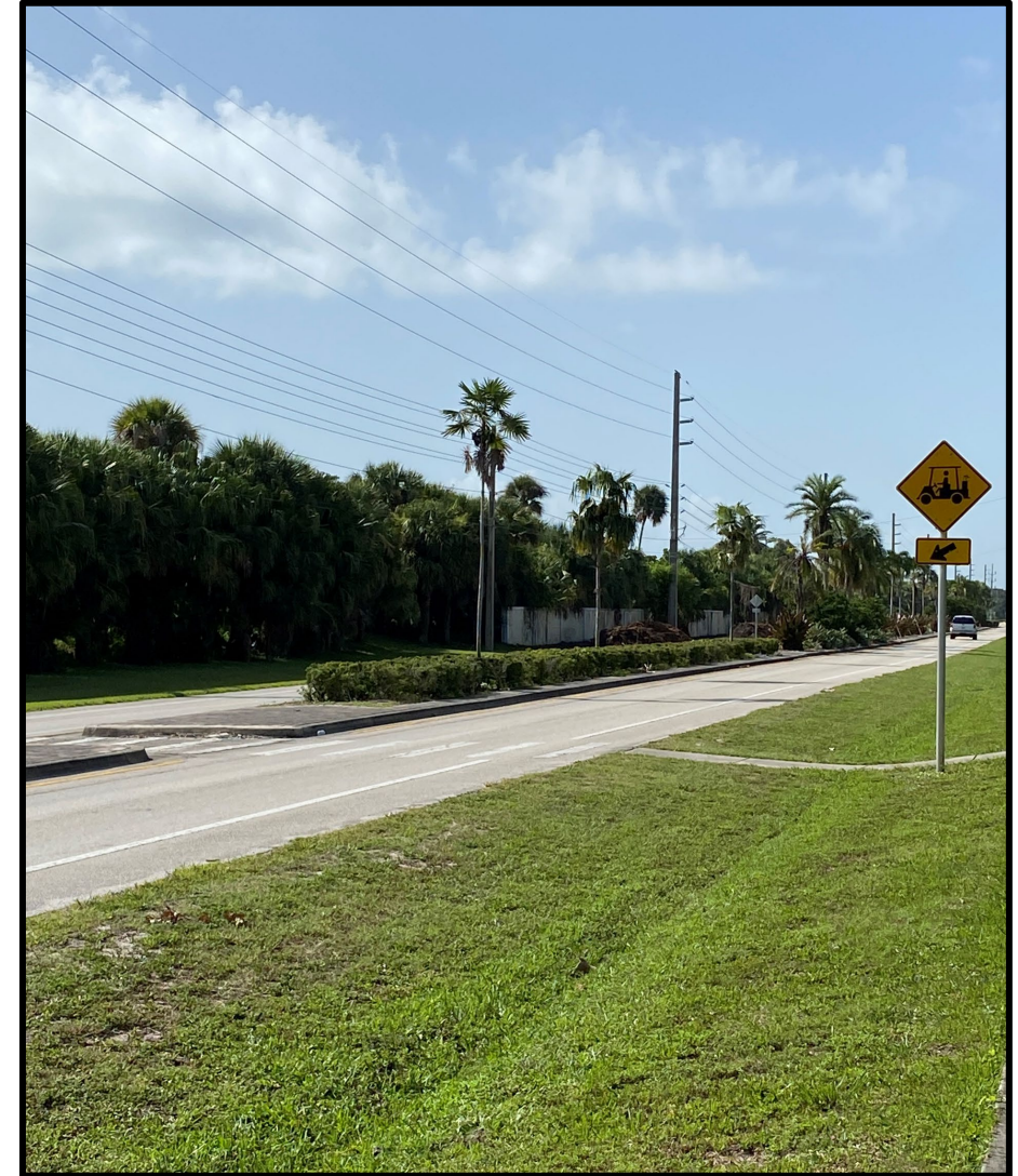
Southbound SR-A1A just south of Bay Drive (pre-construction)
