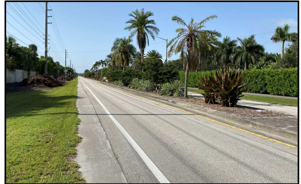
Northbound SR-A1A looking south (pre-construction)
