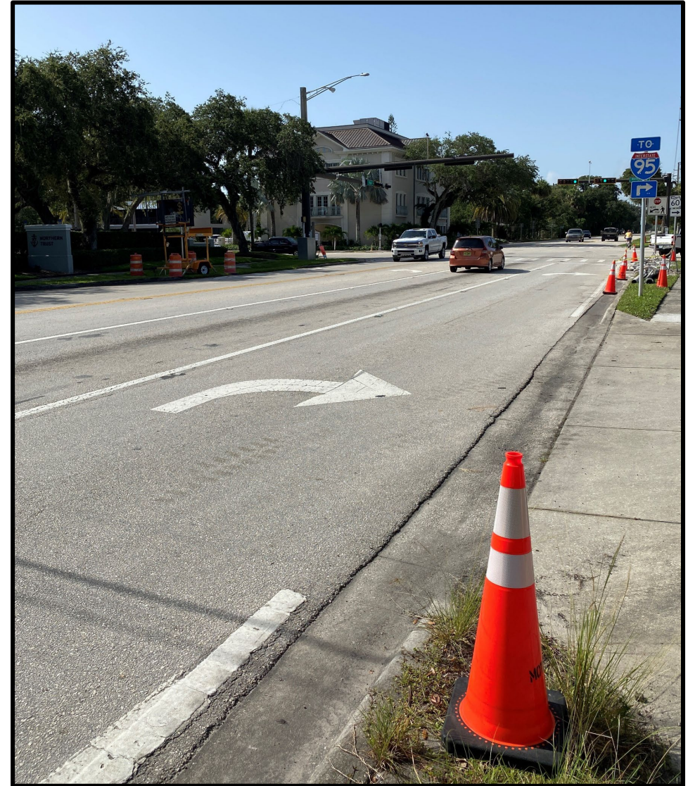
Southbound SR-A1A approaching SR-60/Beachland Boulevard (pre-construction)
