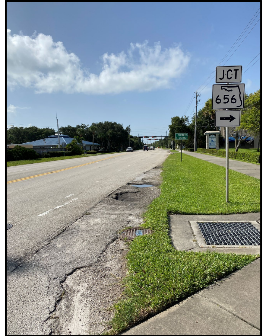
Southbound SR-A1A approaching 17 th Street (pre-construction)
